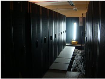
The new computer room is based on the hot aisle/cold aisle principal and can handle IT equipment generating up to 200kW by virtue of six large Stulz air conditioning systems, a battery backed UPS system and a 630kVA standby generator. This level of power supply and cooling equates to over 500 average sized servers.
